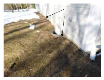
3. Ground elevation is low around the propane tank access cover. Soil elevation should not extend near the cover to allow soil to erode into the tank access opening. Correct grading.
